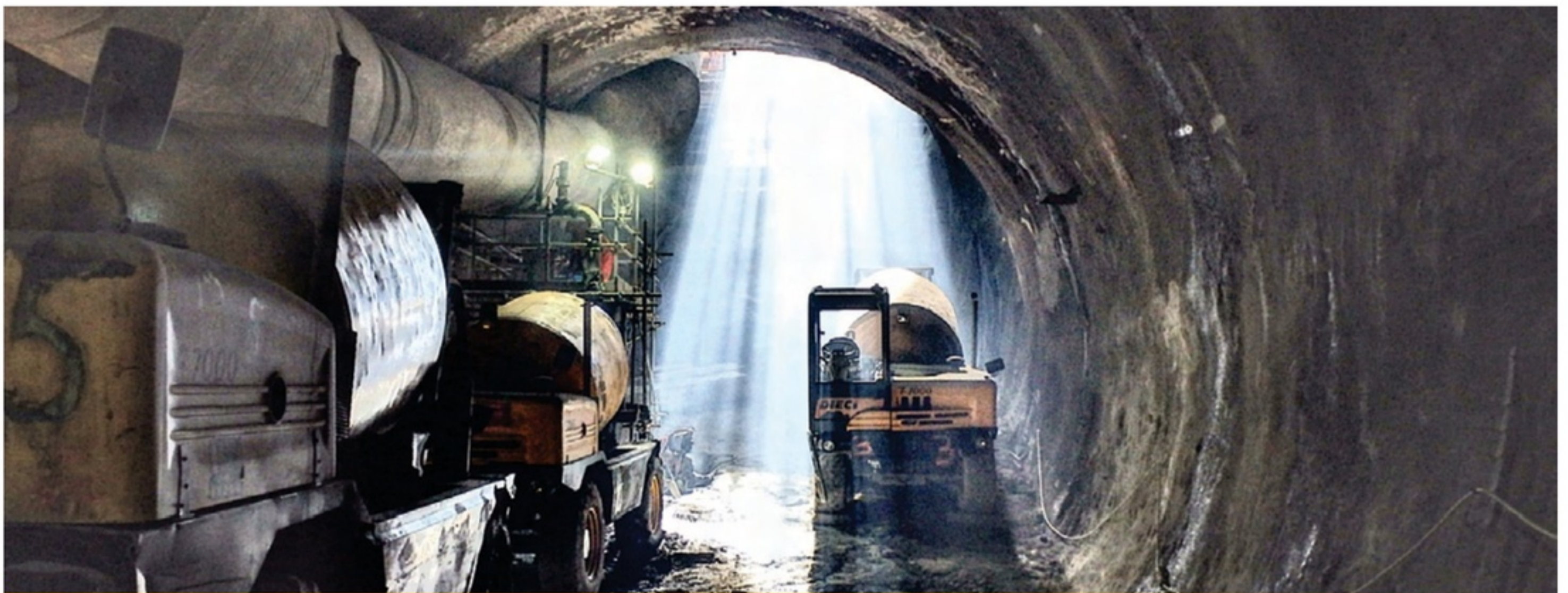
Rockdrain being installed on the concrete lining
